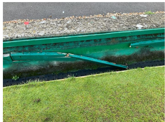
Photo 12: Housekeeping operations around the green include necessary repairs to the ditch impact boards where misplaced steps have caused damage to the wooden batons.
